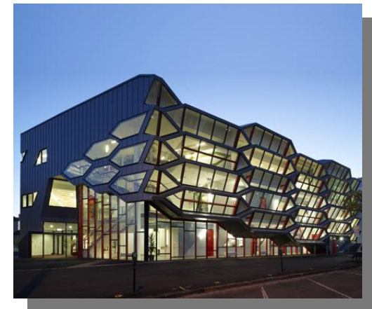
Εικόνα 40: Australian firm Lyons' new campus building for a college in Warrnambool, Australia, has a glazed façade made up of hexagonal apertures tilted down towards the street.
